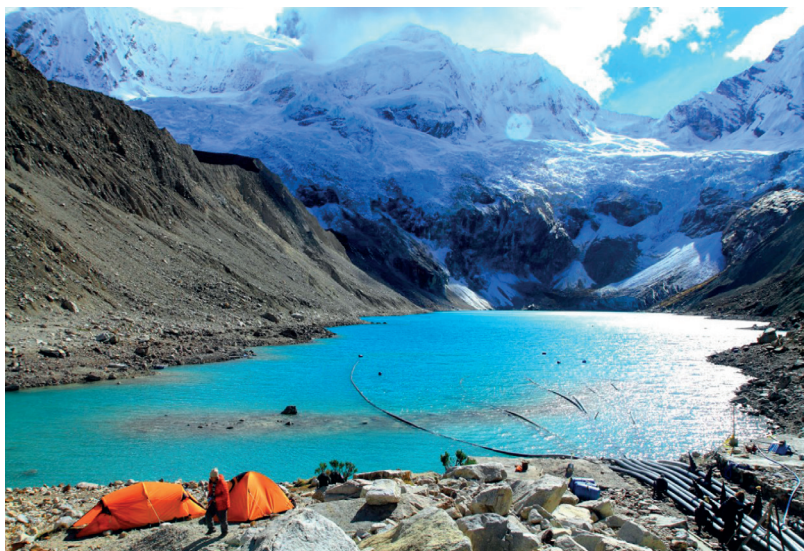
Palcaraju glacier and Lake Palcacocha in 2013, with siphons removing water to reduce the possibility of a GLOF. (Paribesch Pradhan, National Snow and Ice Data Center)
