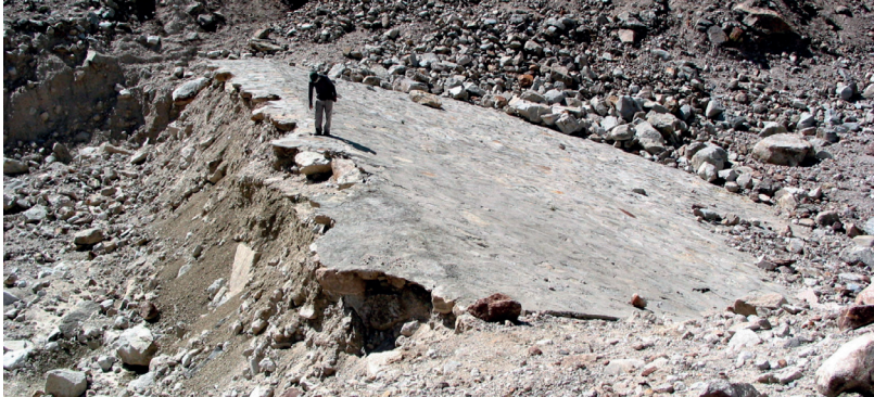
A 2003 photo of Lake Palcacocha's security dam that was partially destroyed when a landslide fell into the lake, creating waves that overtopped the structure. (Mark Carey)
